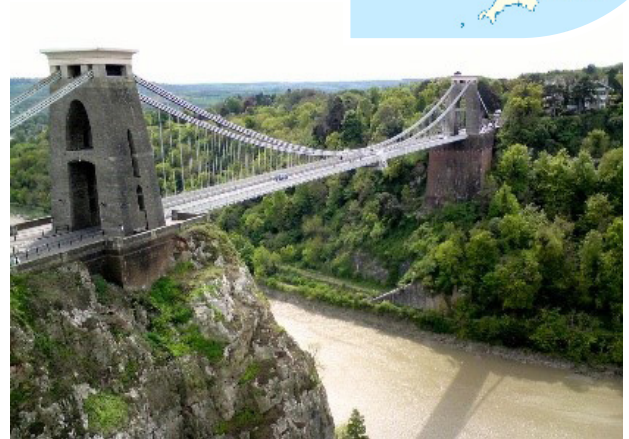
Clifton Suspension Bridge
